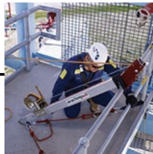
Handrail Recovery Monopole
